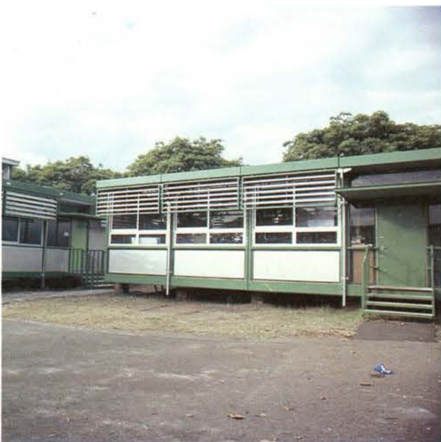
Demountable classrooms at Mosman High School, New South Wales. The ease of transporting and setting up these buildings led to their widespread use to meet short-term fluctuations in the school population. Photograph by Adriaan van der Weel, 1986.
